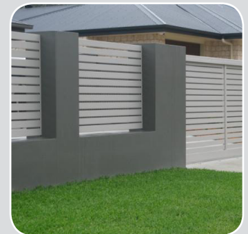
Height blocks façade
